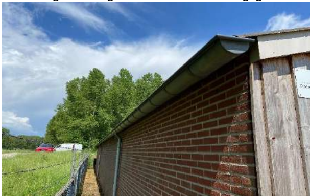
Figuur 1: Dakgoten bebouwing achterzijde (boring 13)
